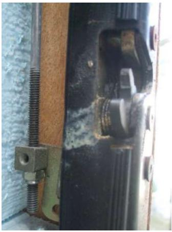
Now put it all back together. Use some contact cement on the gasket at the door corners to glue the gasket back together. You can put the contact cement on before you install the door end and let it dry till it is a bit tacky. Then put the end in place, install the screws, and now press the seal corners together tightly for a few seconds. The contact cement should hold the gasket together almost immediately.
