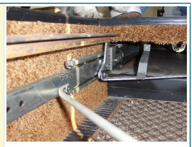
The whole assembly is held in with two screws in the face of the toe kick.
